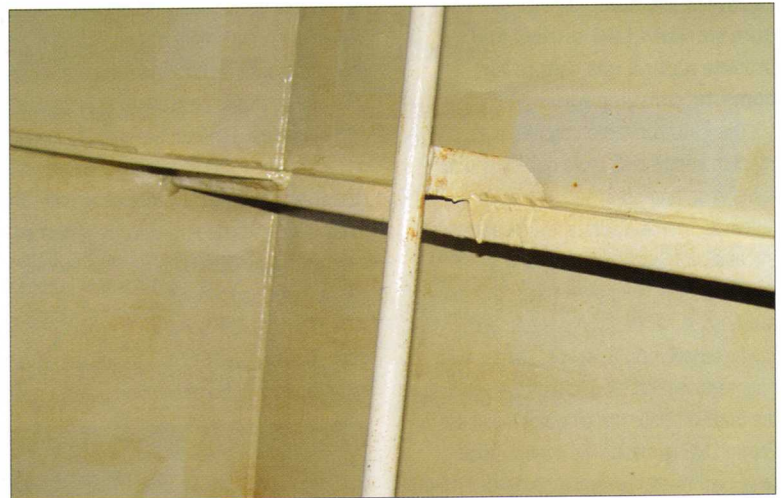
Clean tanks after only one cleansing cycle with the Cytoclean process
